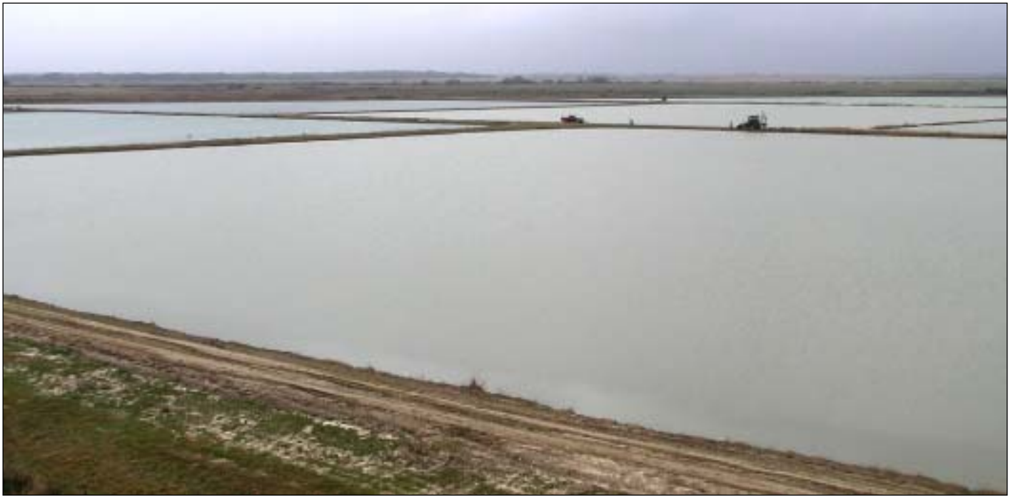
Figure 7. Completed levee ponds.
