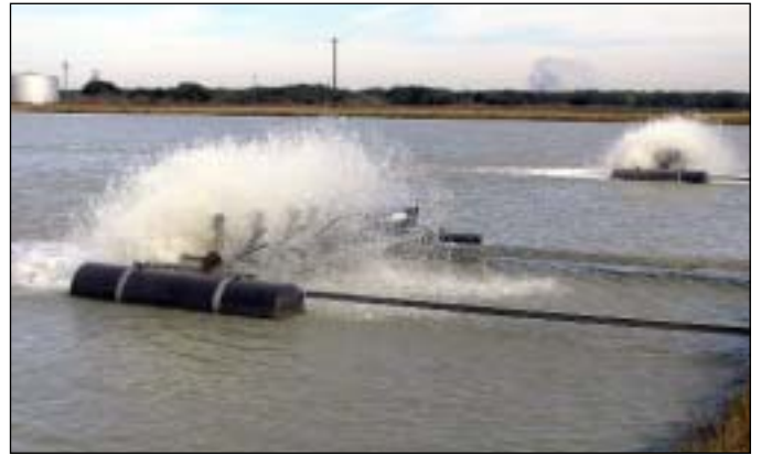
Figure 16. Electric paddlewheel aerators.
