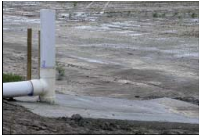
Figure 5. Standpipe drain with concrete balast in a newly constructed pond.
