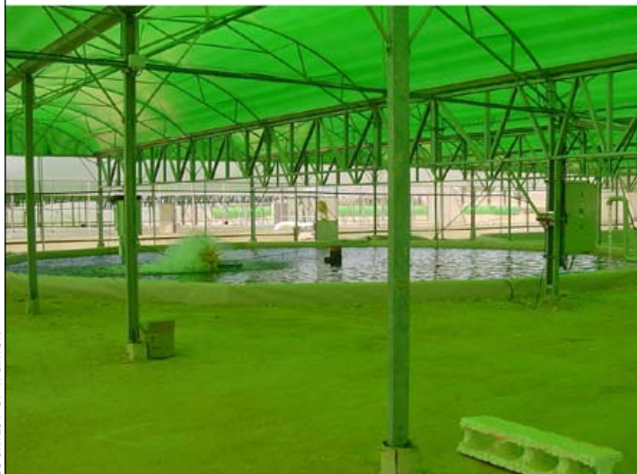
FIGURE 8 Interior of greenhouse containing large tanks for intensive fish culture in Israeli arid Negev. Green plastic is installed to prevent algal blooms in the tanks
