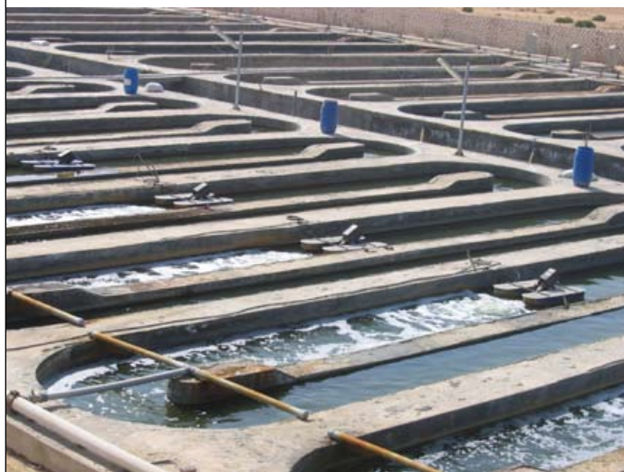
FIGURE 8 D-ended shape tilapia raceway (145 m 3 ) with 2 HP air-injector, in Valley Organic company, El-Beheira Governorate, Egypt
