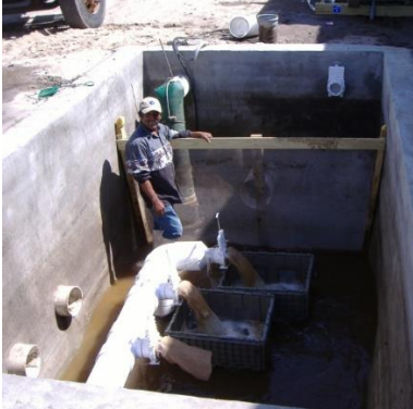
Figure. Drain harvest for juvenile shrimp from the biofloc raceways at Bowers Shrimp.
