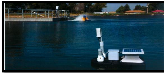
Water monitoring system
