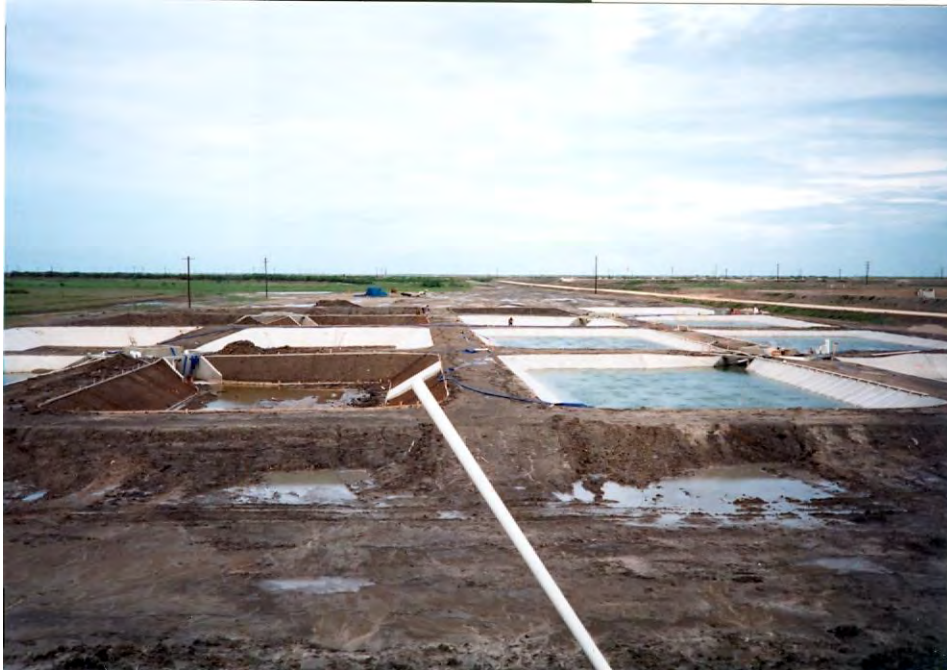
Nursery pond construction at Southern Star, 1990s
